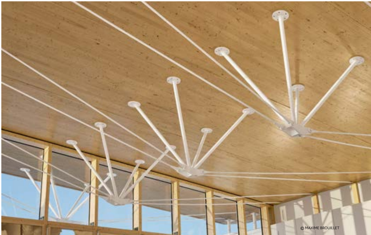
INTERIOR VIEW OF THE CHIBOUGAMAU-CHAPAIS AIR TERMINAL
