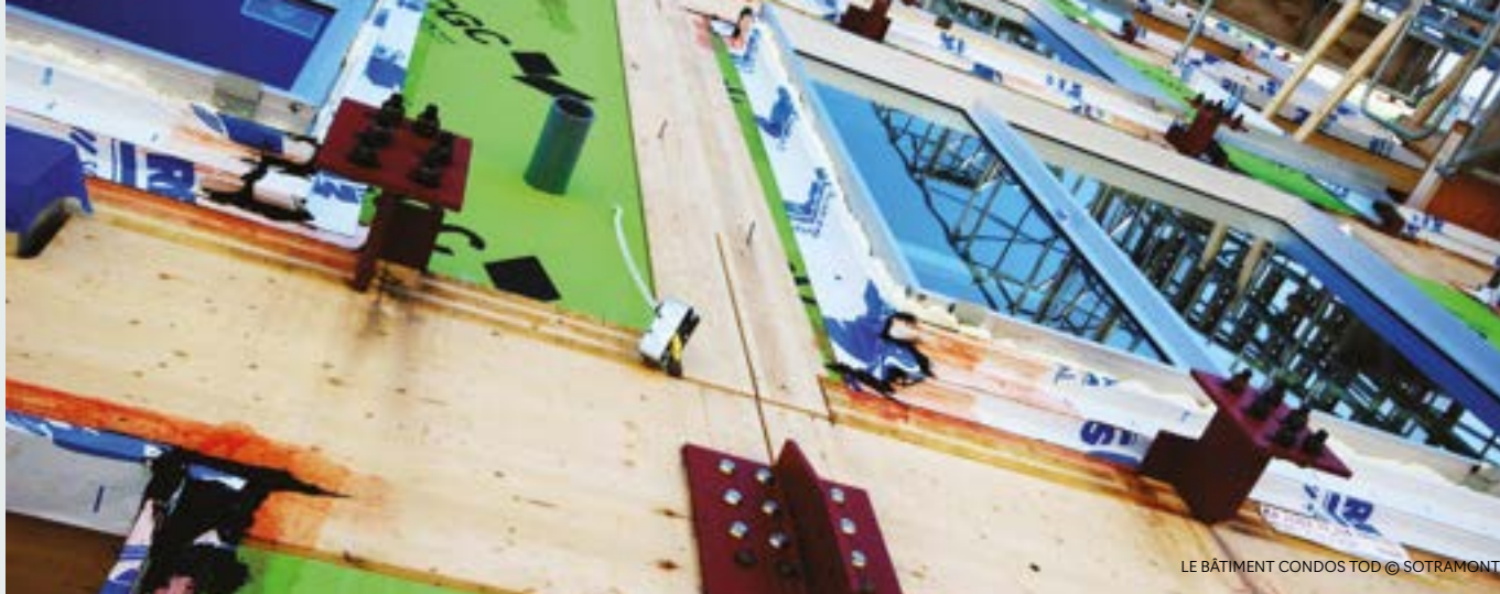
VIEW OF A CLT INTERIOR LOAD-BEARING WALL
